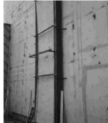
Figure 7 – Full Scale Panel Subjected to Wind Loading During Test
