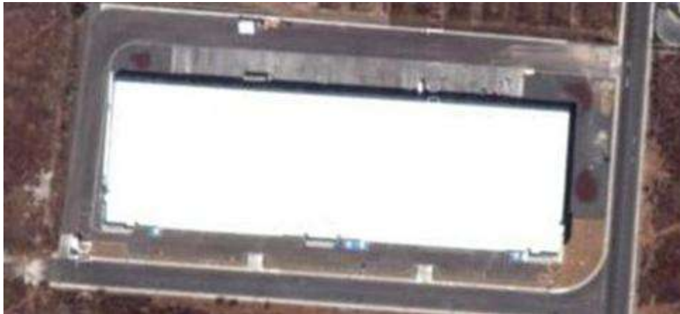
Figure 1: Vesta Inventory III Building Aerial View
