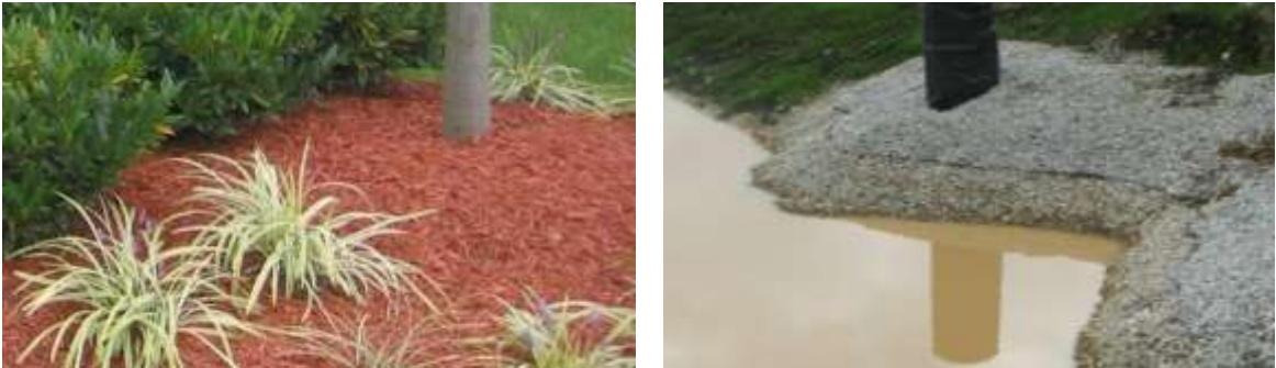
Figure 47: Erosion and sedimentation control – use mulching and temporary seeding
