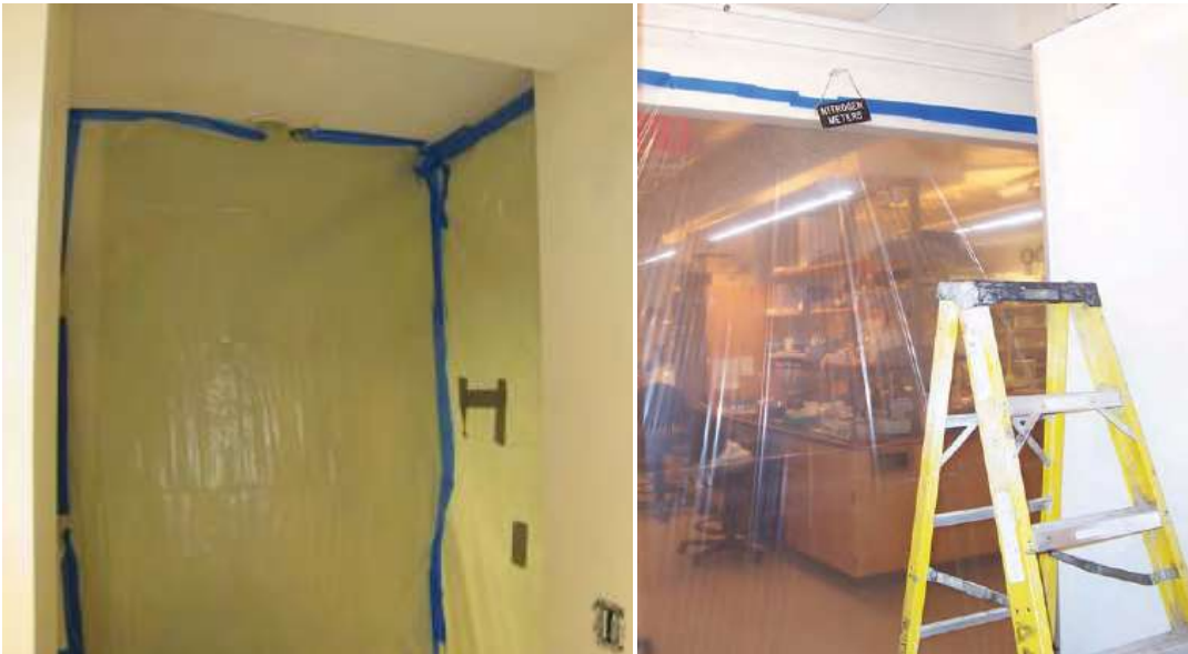
Figure 55: Insolation of construction area from remainder of building (Source: Harvard Green Campus Initiative)
