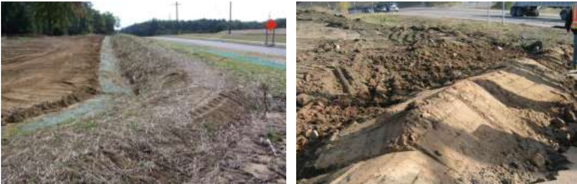
Figure 50: Erosion and sedimentation control – earth dikes
