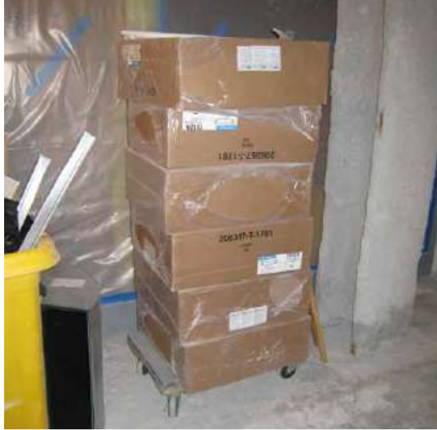
Figure 56: Materials kept off the floor to avoid damage and exposure to moisture (Source: Harvard Green Campus Initiative)
