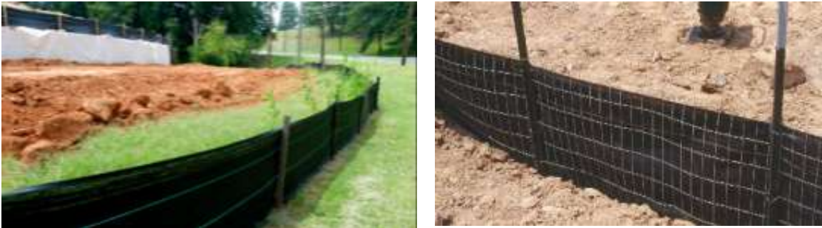
Figure 48: Erosion and sedimentation control – use sediment fences
