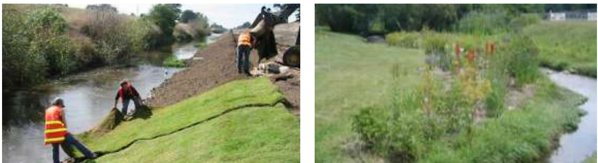
Figure 46: Erosion and sedimentation control – protect and maximize existing vegetation
