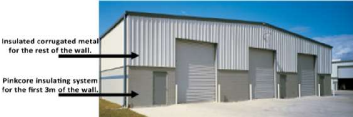
Figure 61: Wall assembly using pinkcore and insulated corrugated panels
