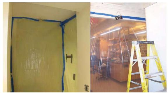
Figure 55: Insolation of construction area from remainder of building
