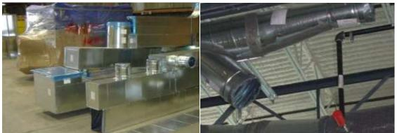
Figure 53:Air quality management plan - HVAC protection (Source: mcaagreen.org)
