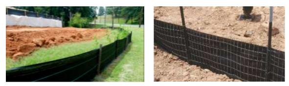
Figure 48: Erosion and sedimentation control - use sediment fences
