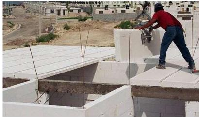
Figure 71: Building construction using Hebel Blocks and Panel Losa Hebel
