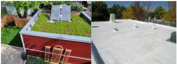
Figure 19: Roofing materials that contibue to heat island effect reduction
