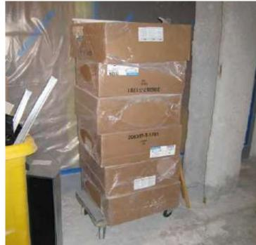
Figure 56: Materials kept off the floor to avoid damage and exposure to moisture (Source: Harvard Green Campus Initiative)
