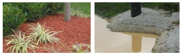
Figure 47: Erosion and sedimentation control - use mulching and temporary seeding
