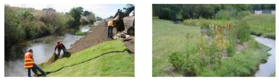
Figure 46: Erosion and sedimentation control - protect and maximize existing vegetation
