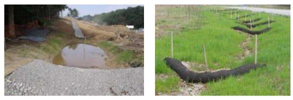
Figure 49: Erosion and sedimentation control - sedimentation basins
