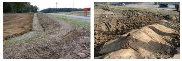
Figure 50: Erosion and sedimentation control - earth dikes
