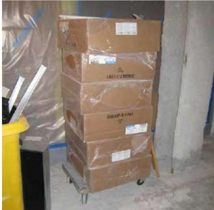
Figure 56: Materials kept off the floor to avoid damage and exposure to moisture
