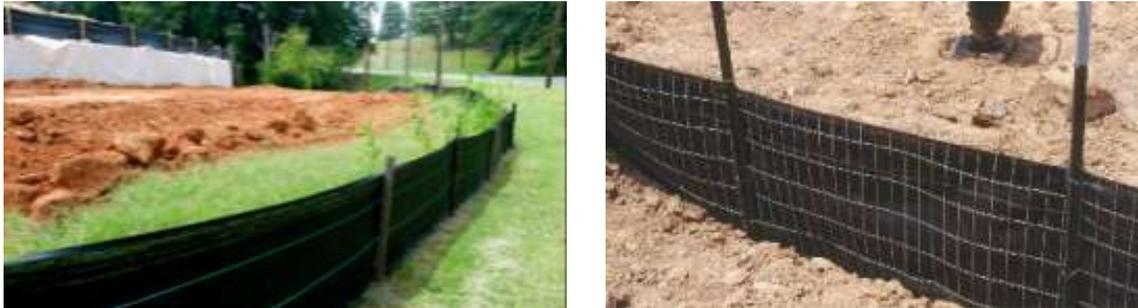
Figure 48: Erosion and sedimentation control – use sediment fences
