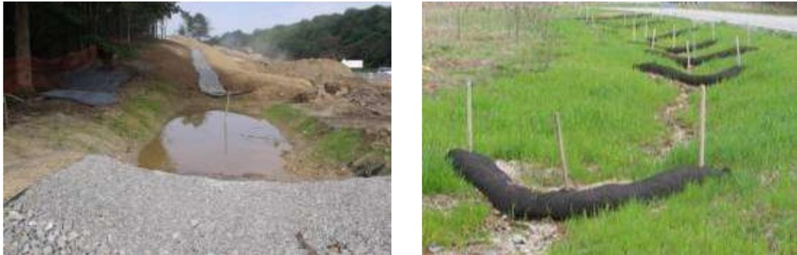
Figure 49: Erosion and sedimentation control - sedimentation basins
