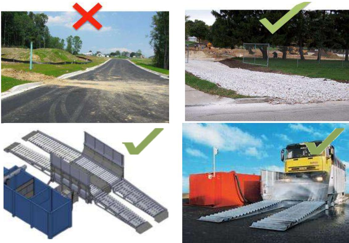
Figure 51: Erosion and sedimentation control – vehicle tracking (Source: aspent.com)
