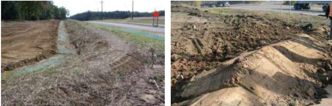
Figure 50: Erosion and sedimentation control – earth dikes
