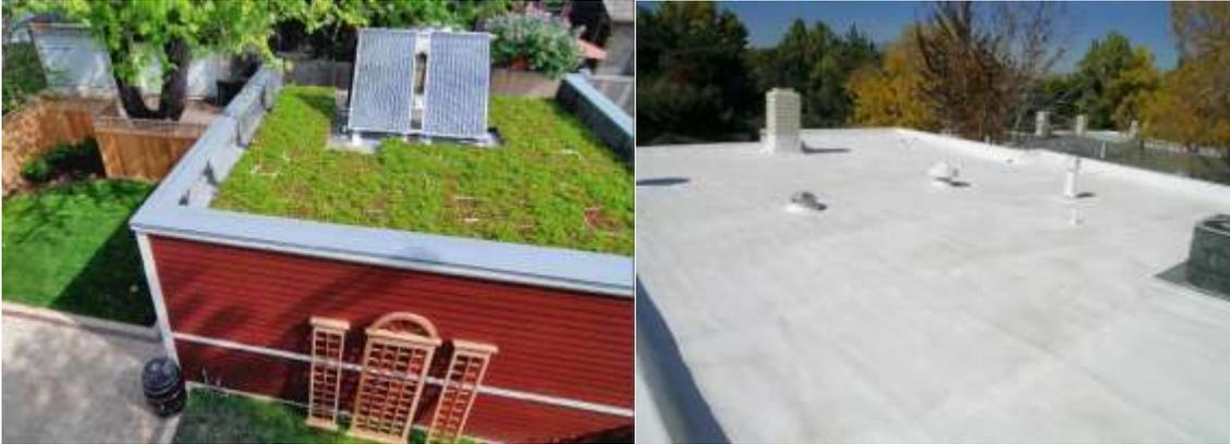
Figure 19: Roofing materials that contribute to heat island effect reduction
